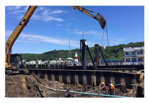
The seven-foot tide change gave workers a small window to install the tie rods. The threaded bar and walers were used in combination to tie the bulkhead wall to the deadman wall. Installation could only be accomplished at the mid-point in the tidal range during daylight hours.
